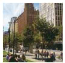
Westin Hotel forecourt, Swanston Street
