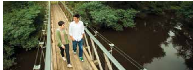
Yea Wetlands swing bridge
